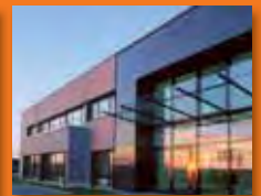
Meisinger facilities at Neuss
